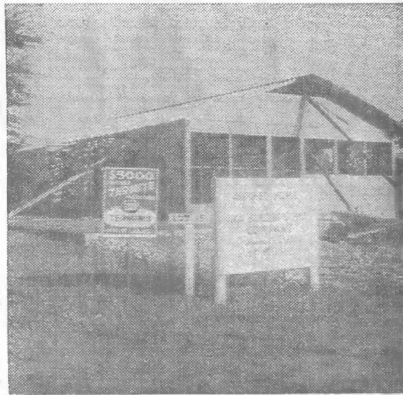
AT RIGHT: Photo at right shows progress made in 12 hours during construction of this Lu-Re-Co. Home. Concrete slab had been completed the previous week. Progress at this stage includes all exterior walls, gables, and roof trusses. Roof decking is in progress in this picture. Note the termite treatment and insurance protection sign.
